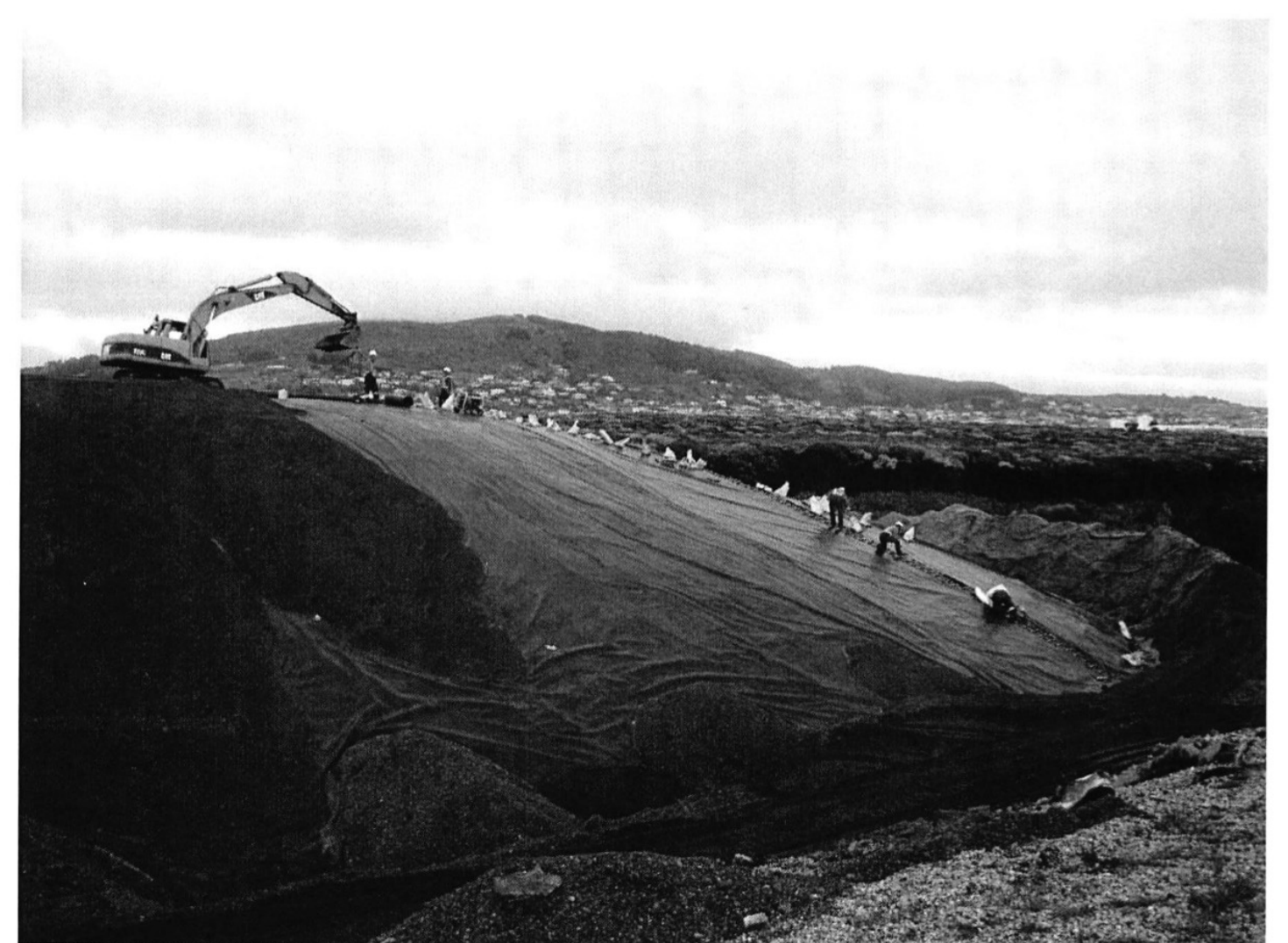
Picture 2 - LLDPE membrane being covered with local pea gravel.
