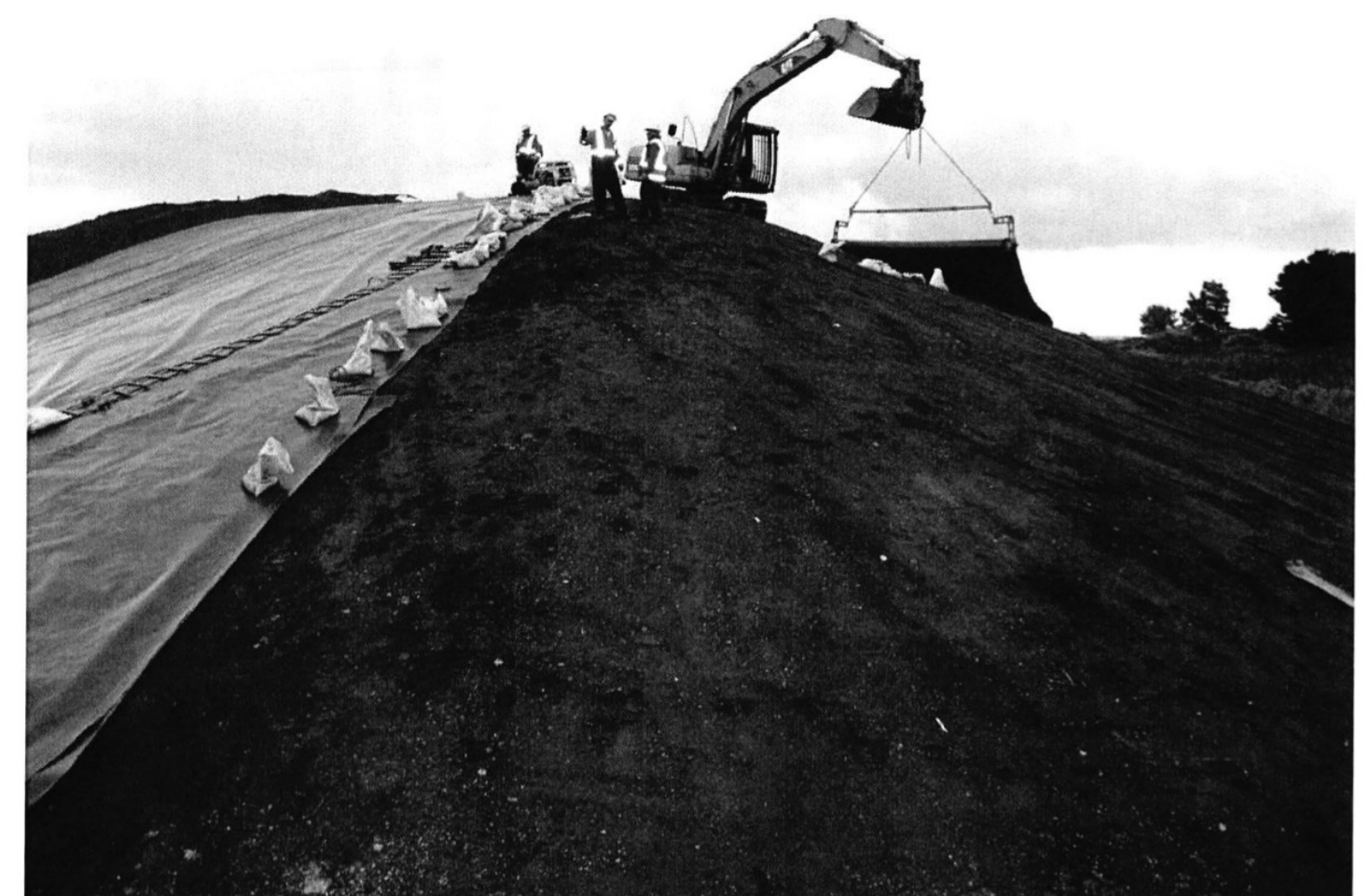
Picture 1 - LLDPE membrane being placed on the Carbon Pile
