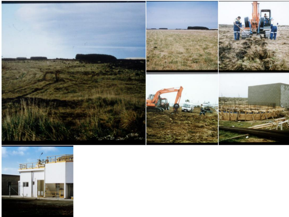
Ecogent supplied design services and subsurface drip irrigation for the Tiwai Point Aluminium Smelter. Refinery wastewater is irrigated under 6 hectares of Department of Conservation lands which to this day it remains the largest industrial SDI installation in NZ. More details coming soon...
